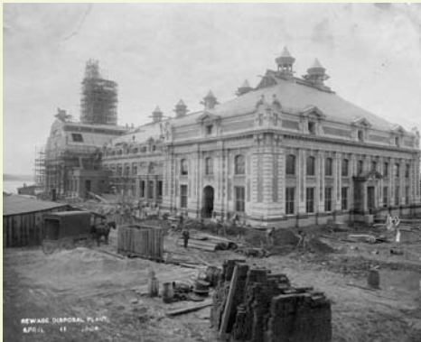
Building the sewage disposal plant on New Jersey Ave., SE, around 1906.
